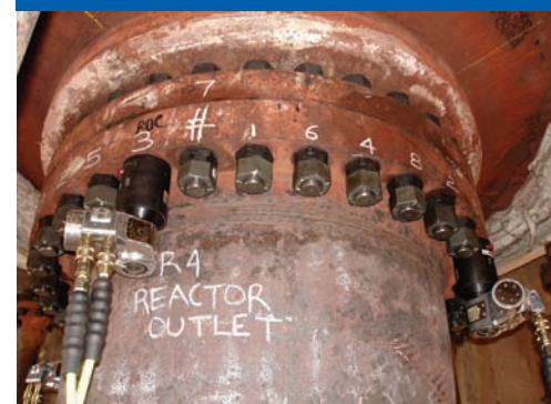
Four HYTORC Avantis™ used hands-free on an inverted application, another benefit of using the HYTORC Washer™.
