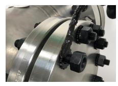
Select proper lubricant to achieve the desired K-Factor for the installation. Apply lubricant to the exposed threads of the bolt.
