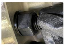
Install the back nut onto the bolt on the rear of the flange and tighten by hand until snug.
