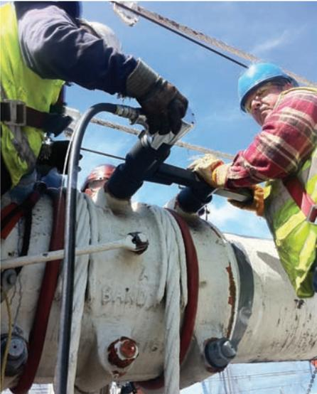
The Torque Gun at work with custom fixture.
