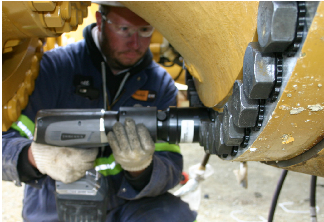
SMART BOLTING USING THE LITHIUM SERIES AND WASHER DRIVER
